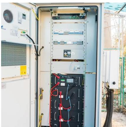
[Outdoor All in One Ess LiFePO4 Air Cooling Batteries Solar Container](#)
