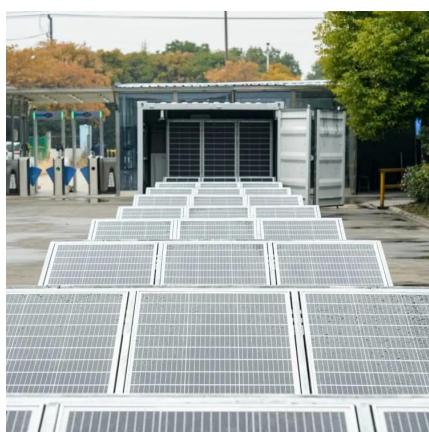
Mar 14, 2025 · Aptech Africa designed, supplied, installed and commissioned the 174.4Kwp Off grid system in South Sudan with a 160kwh battery energy storage with Lithium- ion batteries ...
