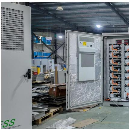
**500kw 800kwh LiFePO4 Lithium Ion Battery Solar Energy System Container**
